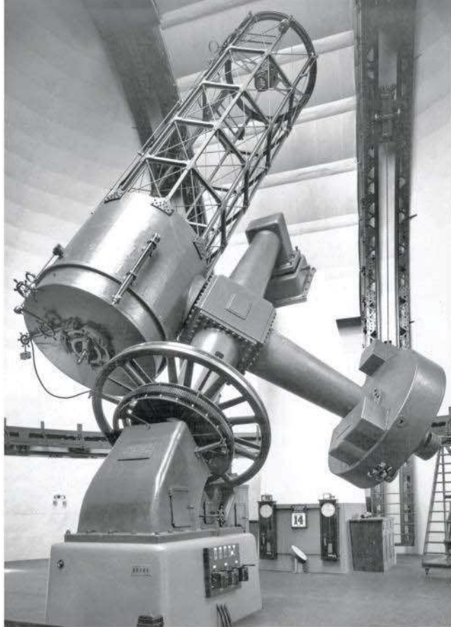
THE UNIVERSE AWAIT Clockwise from left: Assembled and ready for its optics, the 72-inch telescope posed for a formal portrait in the completed dome on July 14, 1917. A four-horse team carefully hauls the truss tube of the giant reflector up a dirt road to the summit of Little Saanich Mountain in 1916—the conclusion of a trip that began in Cleveland, Ohio, where the telescope was fabricated by the Warner & Swasey Company. John A. Brashear pauses with the 72-inch mirror blank at his Pittsburgh factory. Cast by the Saint-Gobain Glass Company of Charleroi, Belgium, the blank was shipped to America shortly before the outbreak of World War I and was sent, finished, to Victoria, British Columbia, in the spring of 1918. ALL PHOTOS COURTESY NRC HAA
