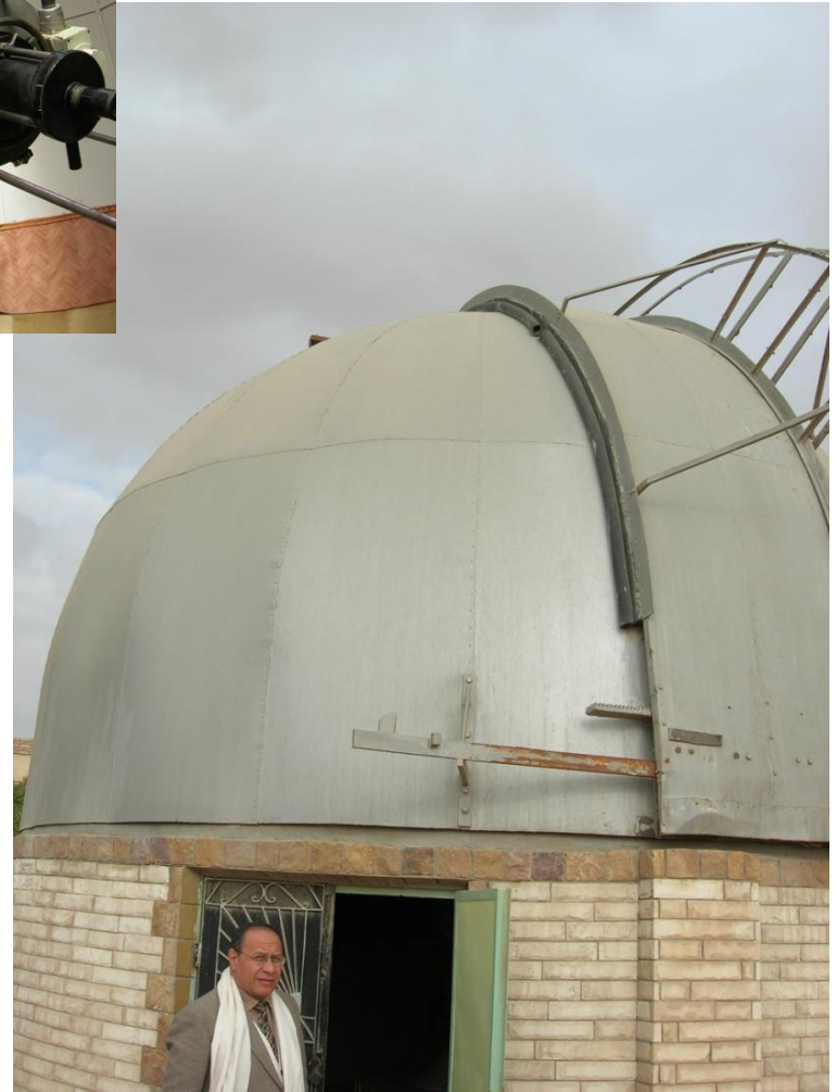
Zeiss-Coude' refractor (6 inch) in Helwan with solar and lunar Camera, and its Dome . Erected in Helwan observatory from year 1946, and still working until now with some modifications
